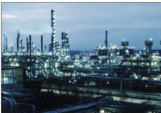
The Wesseling complex in Germany is LyondellBasell's largest manufacturing facility in Europe.
